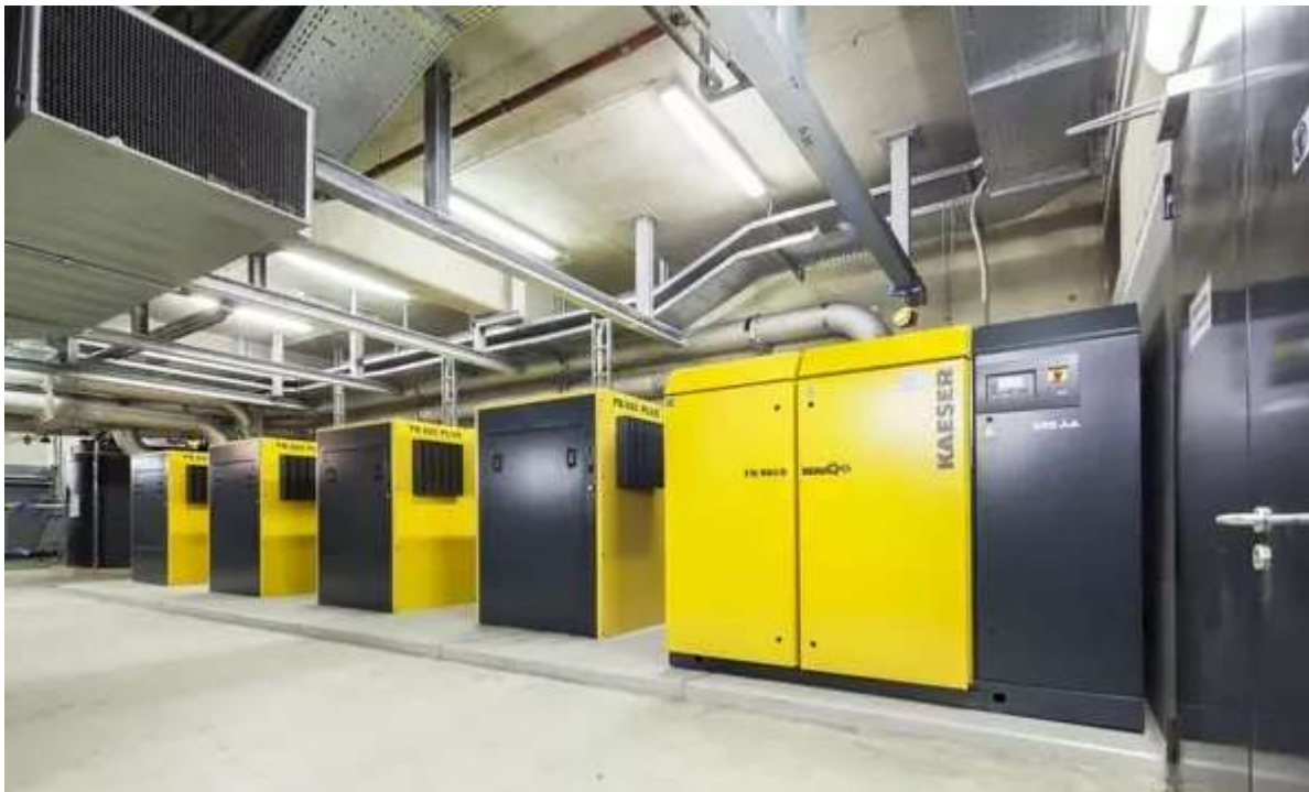
The FBS rotary screw blower in the Treis Karden wastewater treatment plant will replace the previous rotary lobe blower
