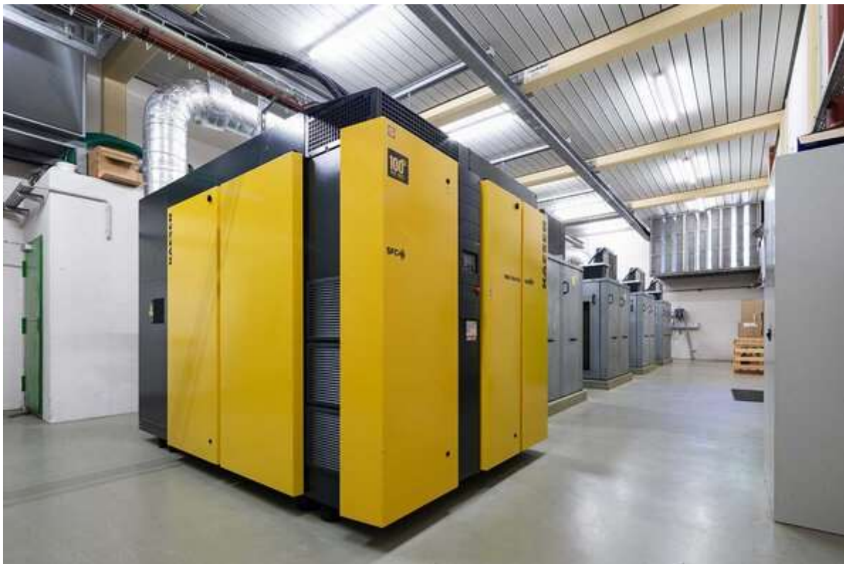
Rotary screw blower from with a max. flow rate of 160 m 3 /min and max. pressure differential of 1100 mbar.
