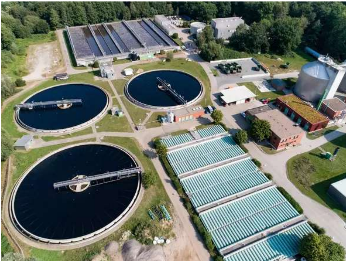
Aeration tanks at the Lüneburg wastewater treatment plant.
